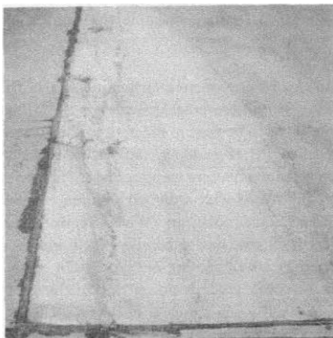
b. State of the damaged area after start of milling
