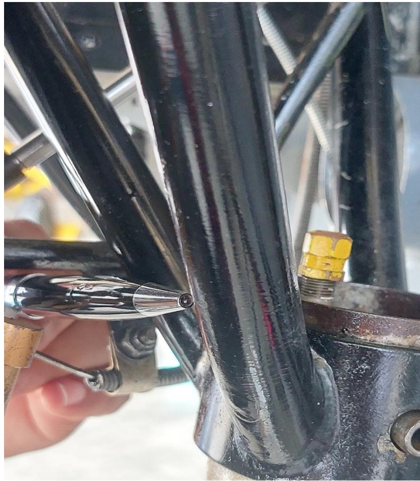
Figure 02: Deformed Engine Mount
